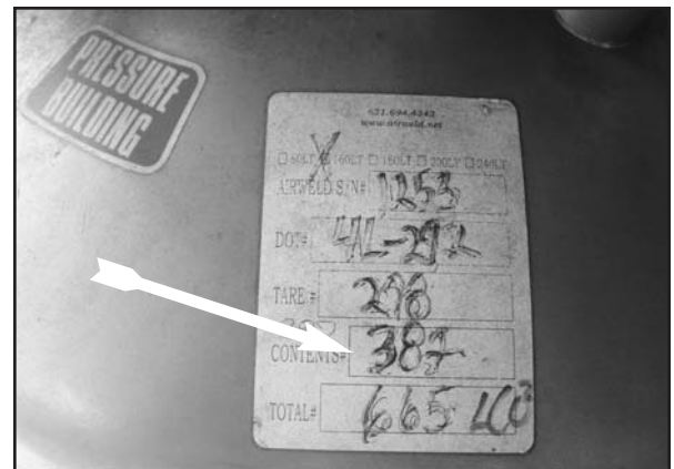
(Far left) Photo #4--Interior installation. The arrow is pointing to CO2 supply line going to the exterior of the building. (Left) Photo #5--Typical exterior installation of Dewar-type CO2 cylinder. (Above) Photo #6--Top of cylinder. Note ID plate attached to the top of the cylinder. The arrow is pointing to the total contents in lbs. when full (387 for this size).
